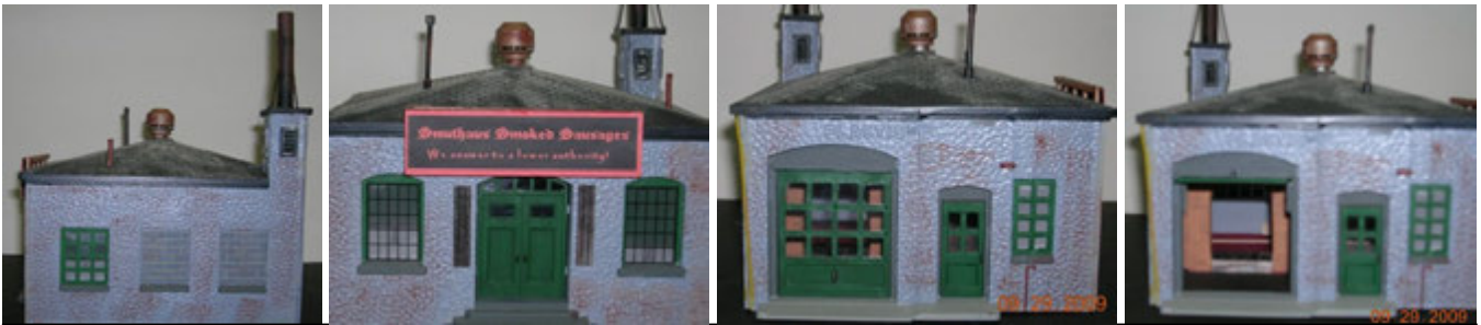
The rear two windows on the right side of the building have been "bricked over" as is common in Brooklyn, NY. (Left photo). The front windows have been replaced by the current occupants as well as the "holes" where the lamps existed have been "boarded up". The sign over the door reads Smuthaus Smoked Sausage / We answer to a lower authority. (Center left photo). The two pictures on the right show the back of the building with the truck door closed.
